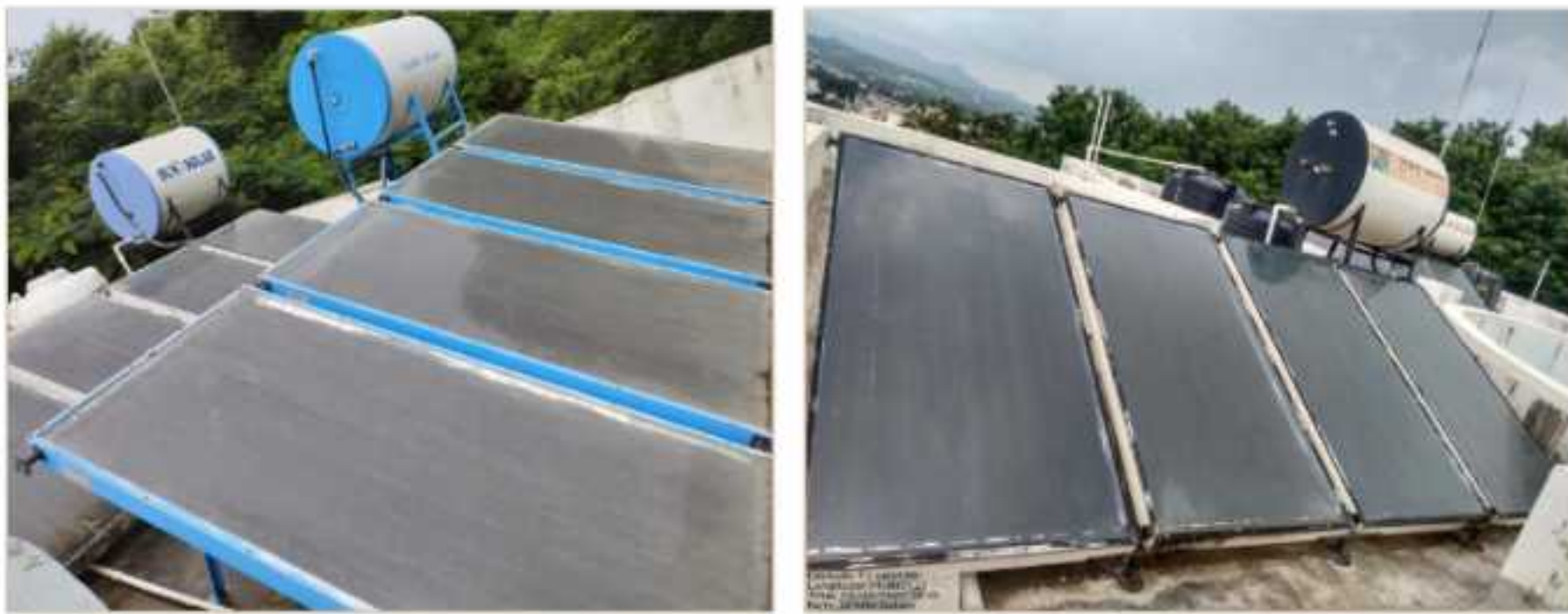
Investigative parameters – Energy Management – Solar hot water heater systems in the premises
