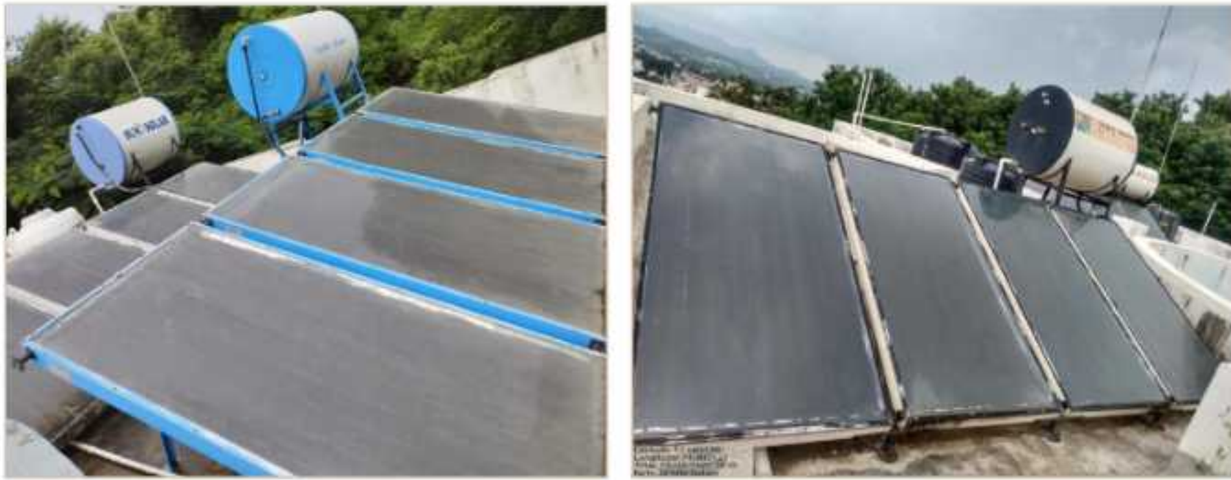
Investigative parameters – Energy Management – Solar hot water heater systems in the premises
