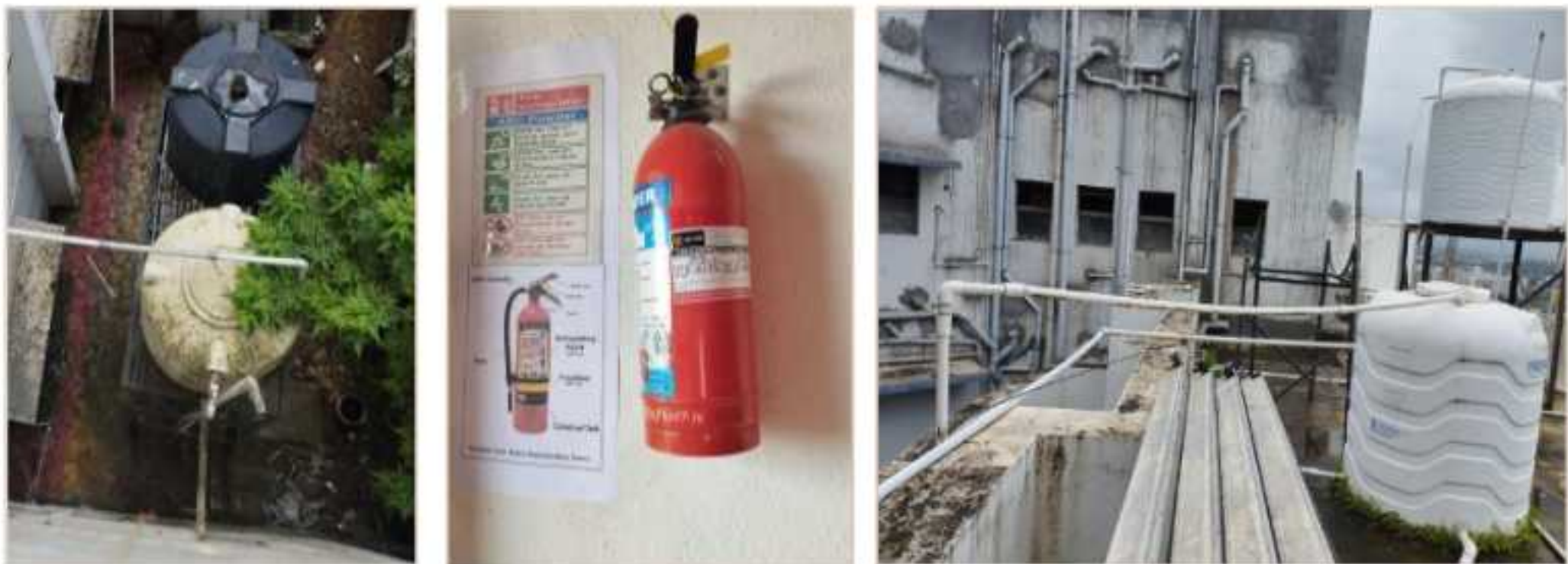
Investigative parameters – Infrastructure facilities in the premises
