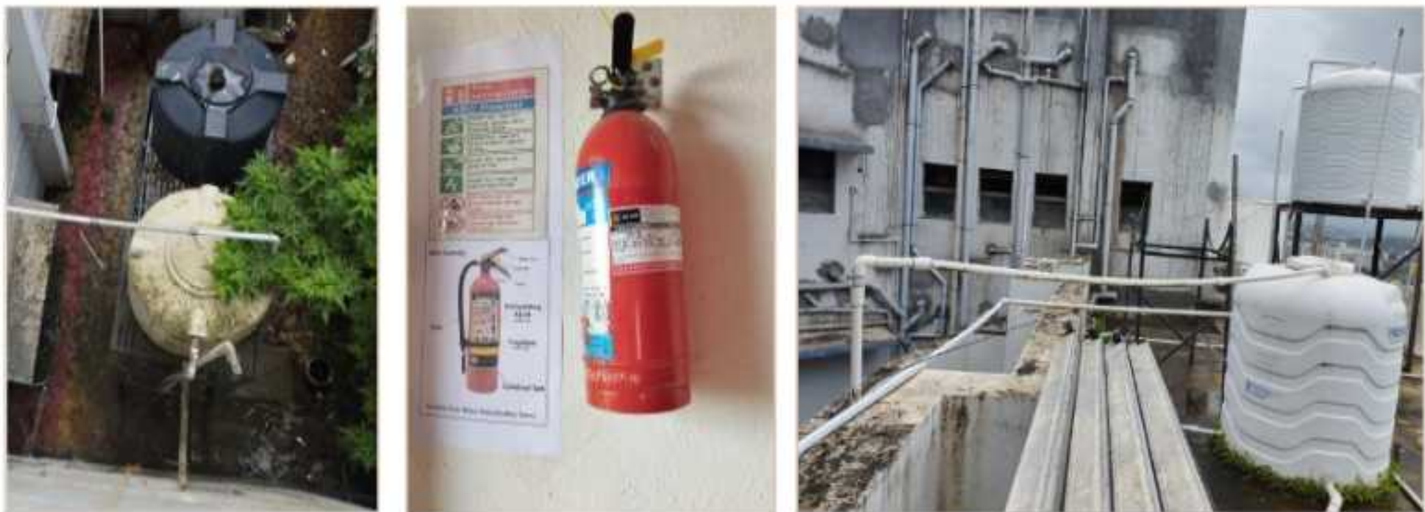
Investigative parameters – Infrastructure facilities in the premises
