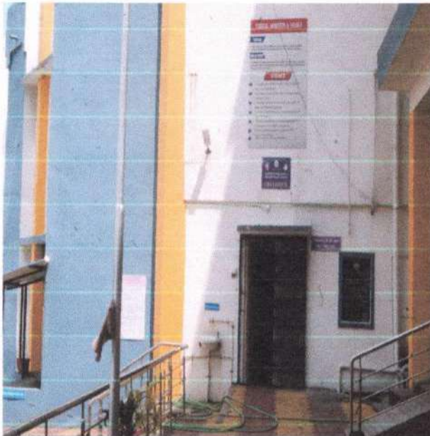
Ladies Hostel Building
